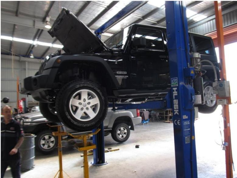
Raise vehicle and support front axle with axle stands.
