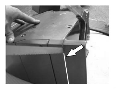
( E ) Place the center consol over the Safe (Item 1) as show, lining up the holes in the side of the center consol with the mounting points on the Safe. Secure the consol to the Safe using four M5 x 25 Button Head Bolts and four M6 x 16 Flat Washers (Items 4 & 5).
