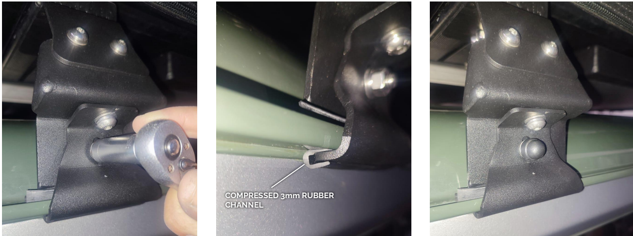
Figure 7 : Completing gutter mount fitment
