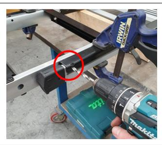
1.3) Locate the horizontal hole in U-bracket on the outside RH side of the ladder and drill this out to 8mm.
